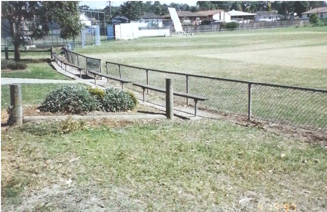
Photo of the original steel post and chain wire fence.
