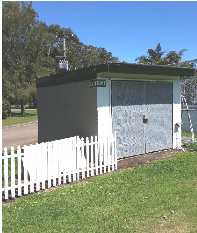
The wicket soil shed, photo taken 26 September 2016. The steel mesh gates were provided by cricketer Cameron Young and the cricket club paid for the installation.
