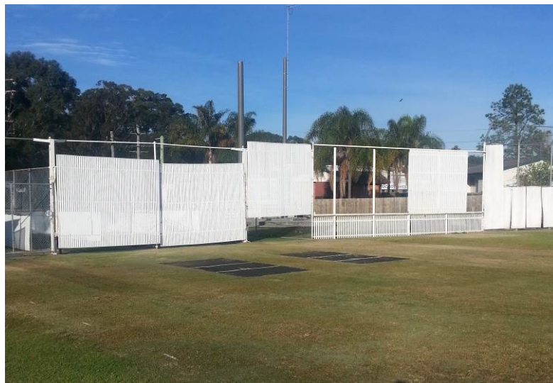
Photo of the sight screens at the southern end of the ground on 3 June 2016. Note the second gate has dropped and the cricket club has new bigger hinges to install to lift the gate.
